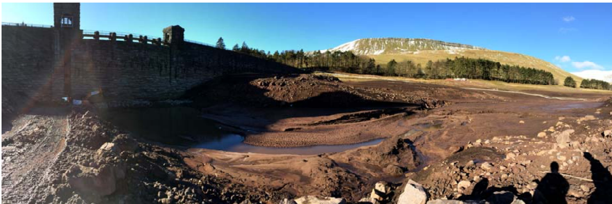
Reservoir basin – silt
