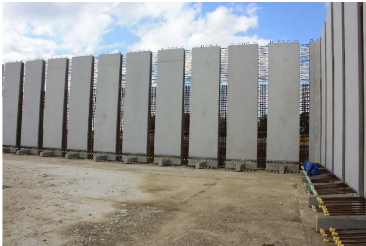
Grafham treated water reservoir
