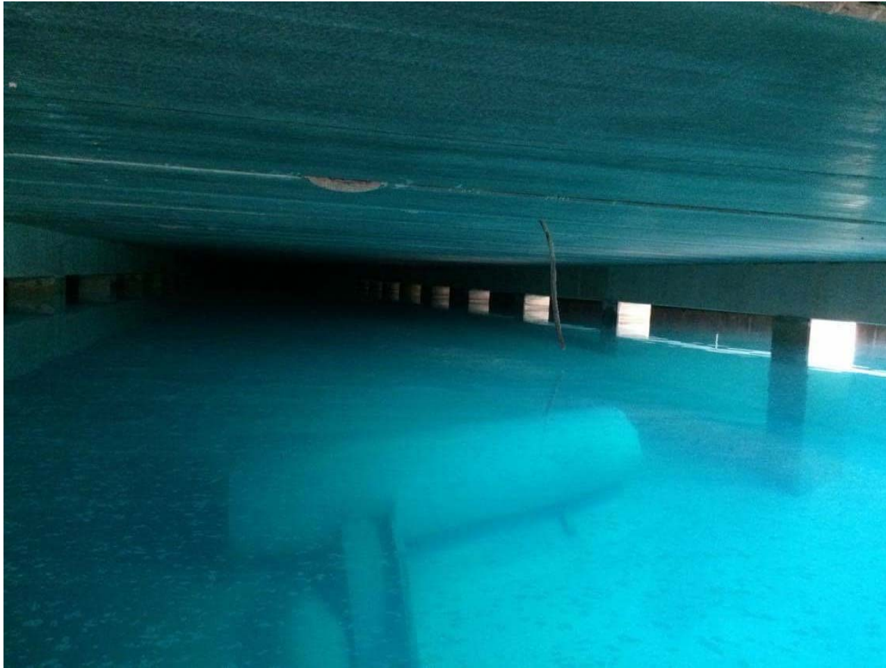
Reservoir under water test
