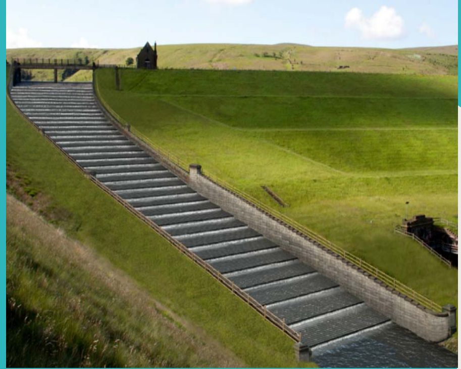
Improved Spillway - Complete
